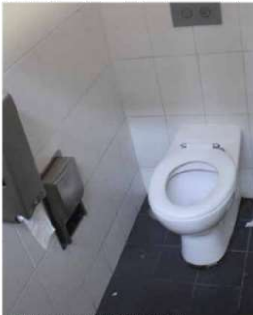
Toilet with concealed cistern, porcelain pan and stainless steel fixtures.
