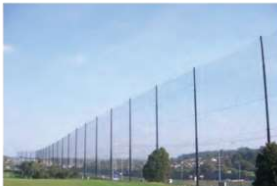
Low visual impact, high safety fence. Kevlar reinforced mesh, timber post supports.
