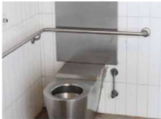
The toilet has a concealed cistern and stainless steel fixtures and fittings.
