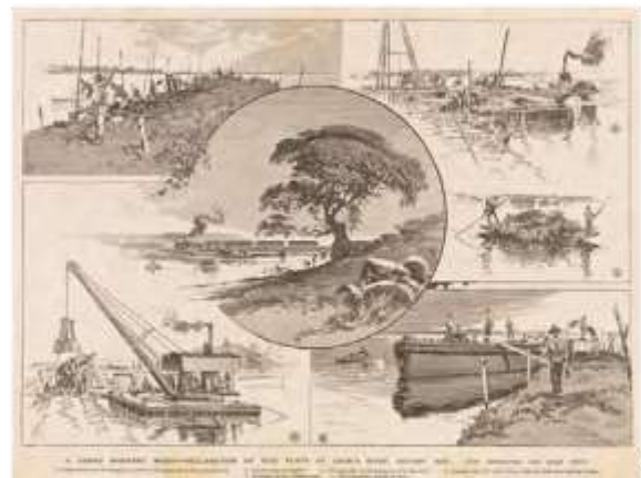
Reclamation of Cooks River 1888, (Showing processes involved in reclaiming mud flats) Source: State Library of NSW
