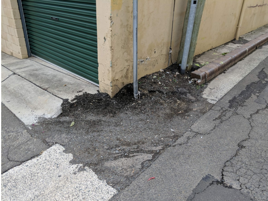
Figure 5.2: Kerb Runover at Farrow Lane
