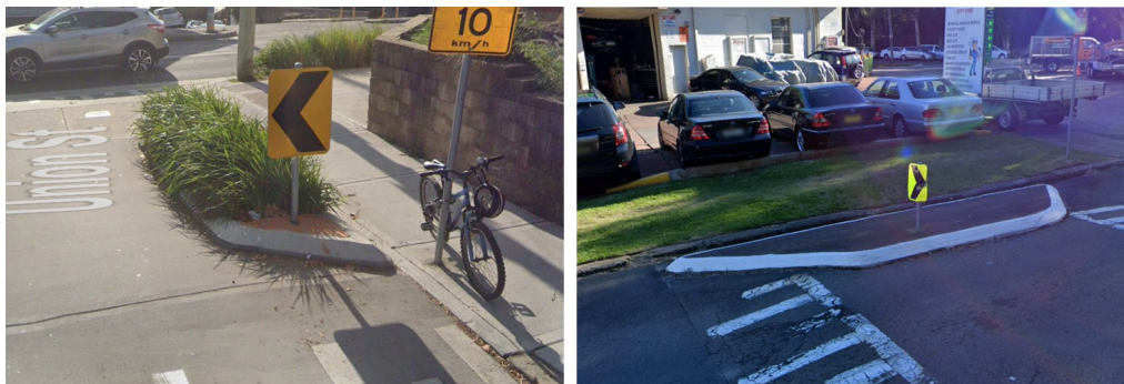
Figure 12.2: Kerb Blisters – Landscaping (left) and Standard (right)
