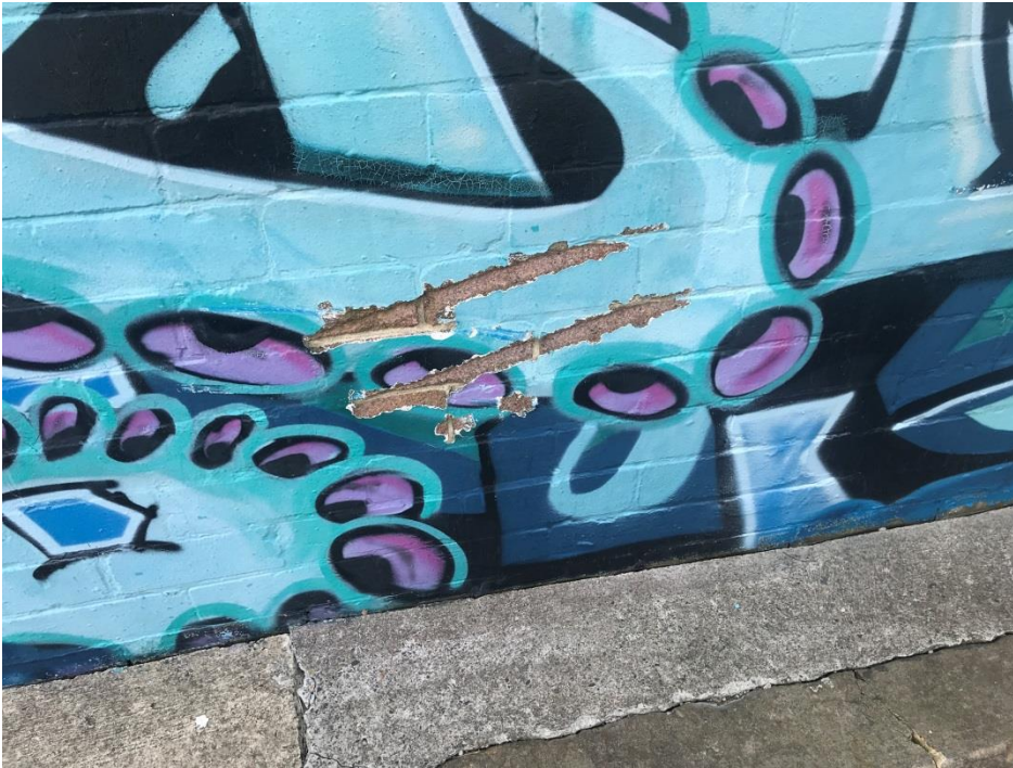
Figure 5: Damage to building on northern side of laneway (potentially due to camber)
