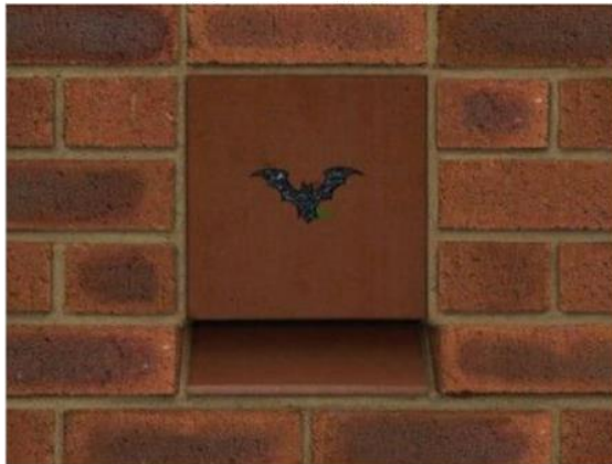
Example of a bat box integrated in a brick facade
