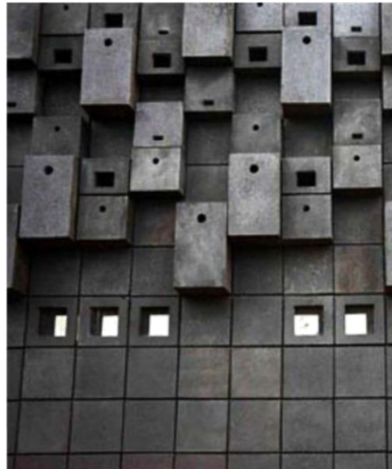
Example of roosting boxes integrated in architectural facade of building
