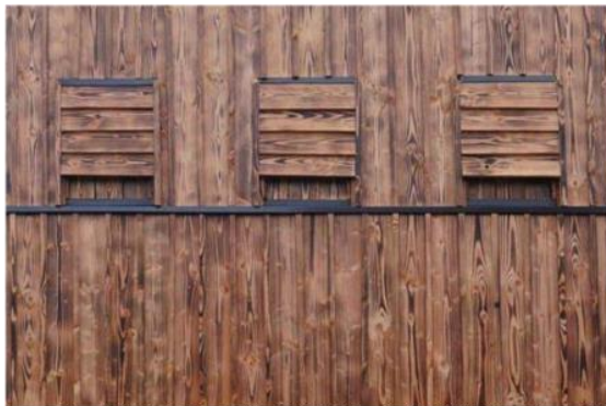
Example of a bat box integrated in a timber facade
