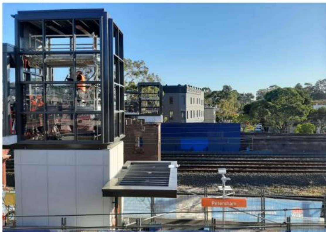
Above: Glass panels being installed in the new lifts at Petersham Station in May.
