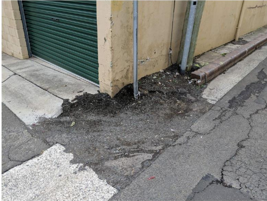
Figure 5.2: Kerb Runover at Farrow Lane
