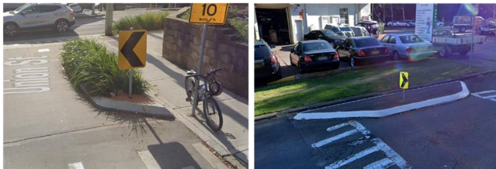
Figure 12.2: Kerb Blisters – Landscaping (left) and Standard (right)
