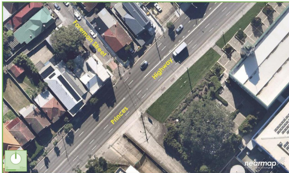
Figure 7: Intersection of Princes Highway and Foreman Street
