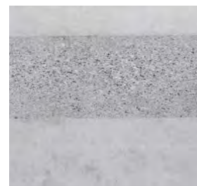
Sandblasted concrete pavement
