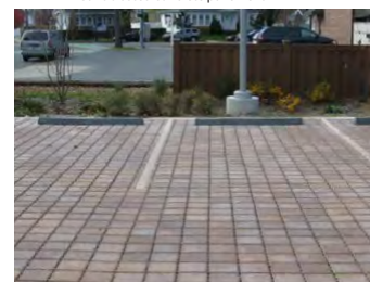
Permeable paving
