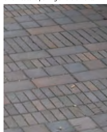
Mixed format brick feature paving
