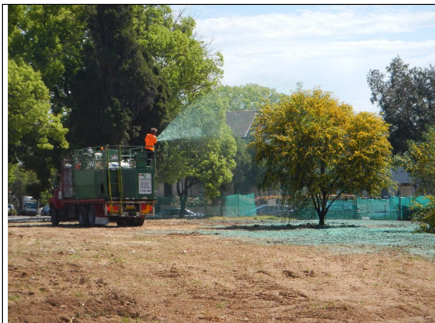
Site Photograph 10: View looking north-west – application of spray grass
