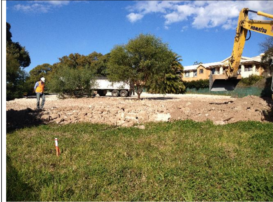
Site Photograph 9: View looking south-east – site during spreading of sandstone
