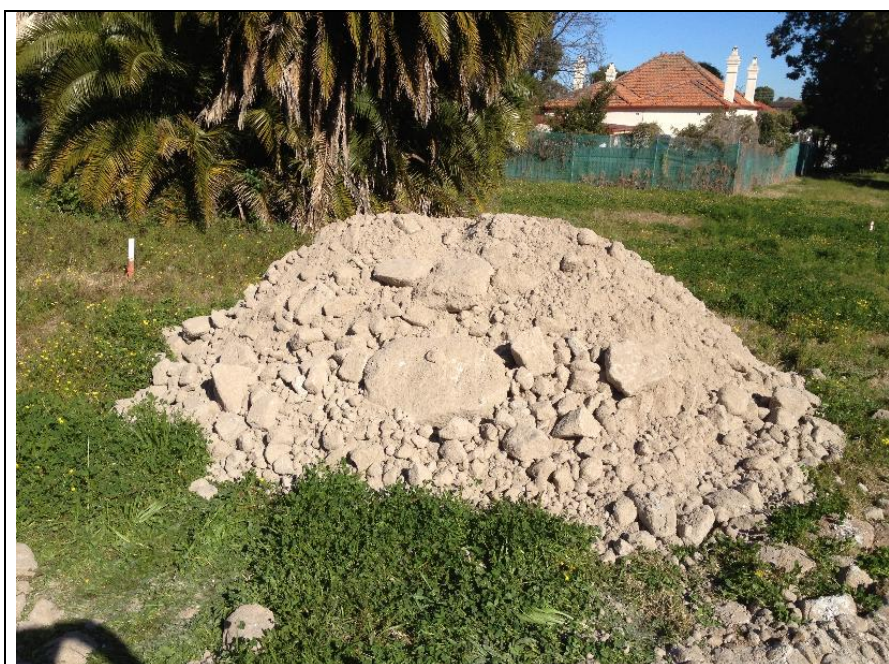
Site Photograph 2: View looking west - imported sandstone and peg marking depth of cap required
