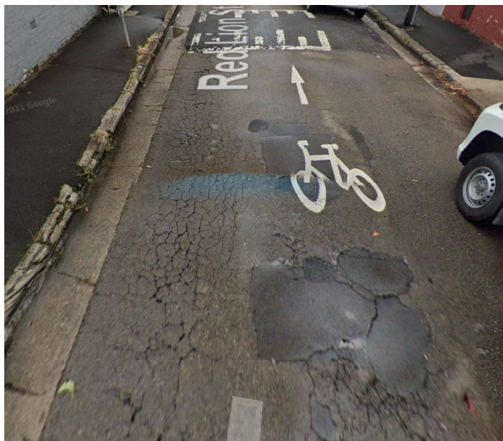
Figure 13 – Major cracking and patchworks along Red Lion Street (Google Maps 2021)
