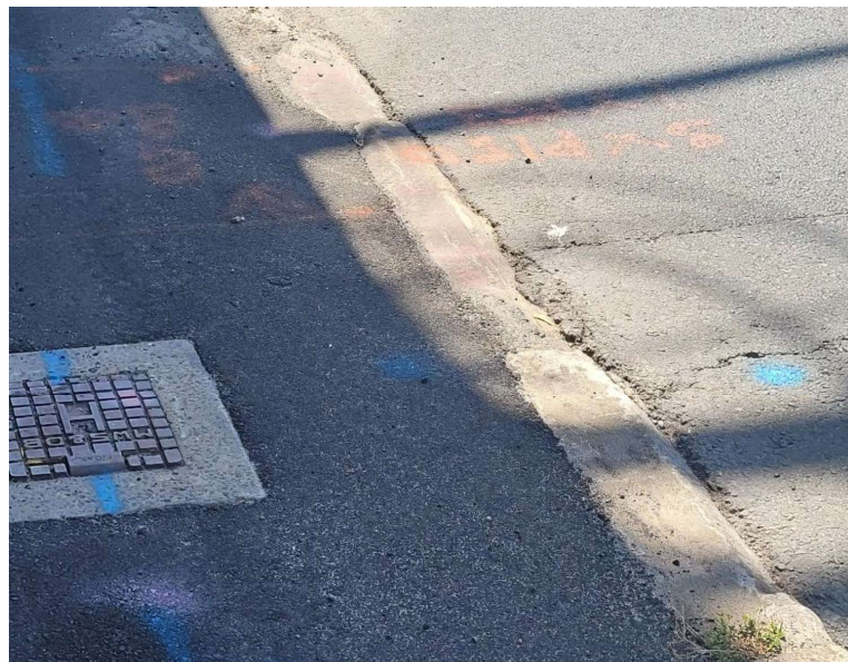
Figure 2: Image showing the depressed pavement along Victoria Road.
