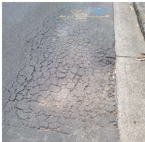
Figure 12 – Crocodile cracking and pumping of fines along Belmore Street
