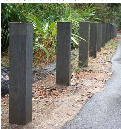
Low impact bollards to protect areas of parkland from vehicles. 5
