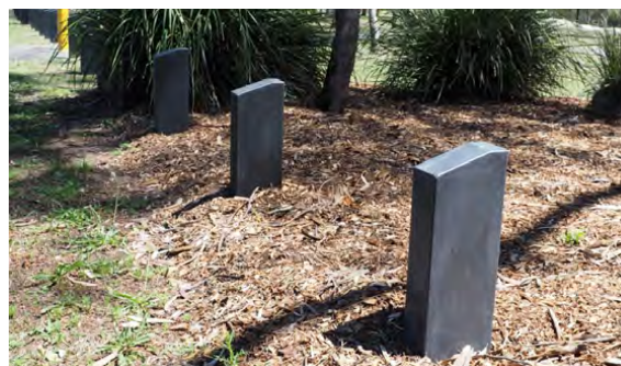
Low impact recycled lumber bollards to protect areas of parkland from vehicles 1
