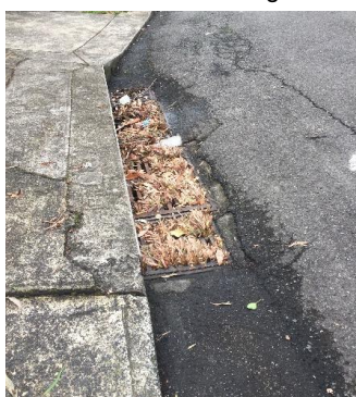
Photo 1: Debris blocking drains on Station Street
