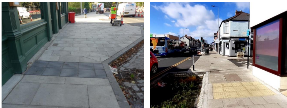
Figure 8: Non-standard layout/style of tactile paving
