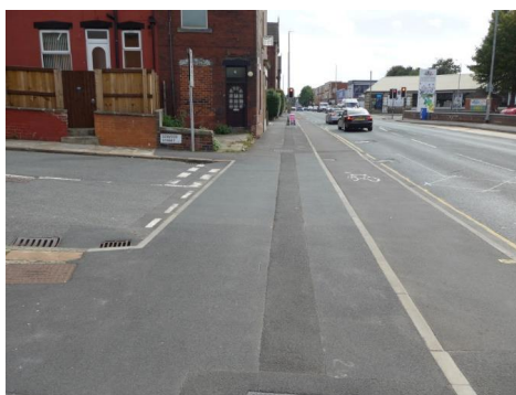
3) Little carriageway-footway contrast. Drivable space at carriageway level. Interpreted as continuation of footway?
