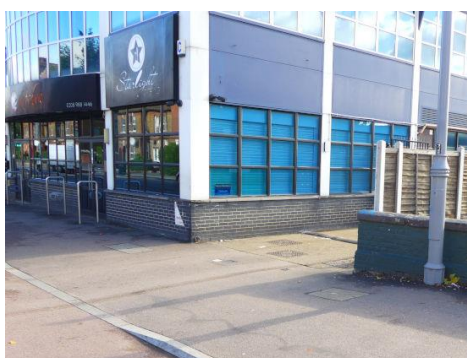
5) Private entrance over footway. Frequent access by large vans. Footway drops to carriageway level.
