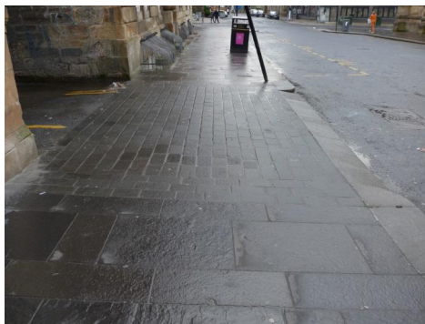
1) Footway appears to continue in an unambiguous way. Drivable space at footway height. Steep access ramp.
