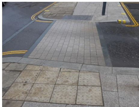
2) Drivable space at carriageway height, but significant contrast with carriageway surface and similarity to footway surface.
