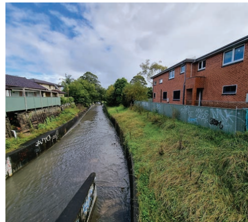
View from Church Street looking upstream, showing approx. 2m open space on the eastern side of the channel and 5-6m on the western side
