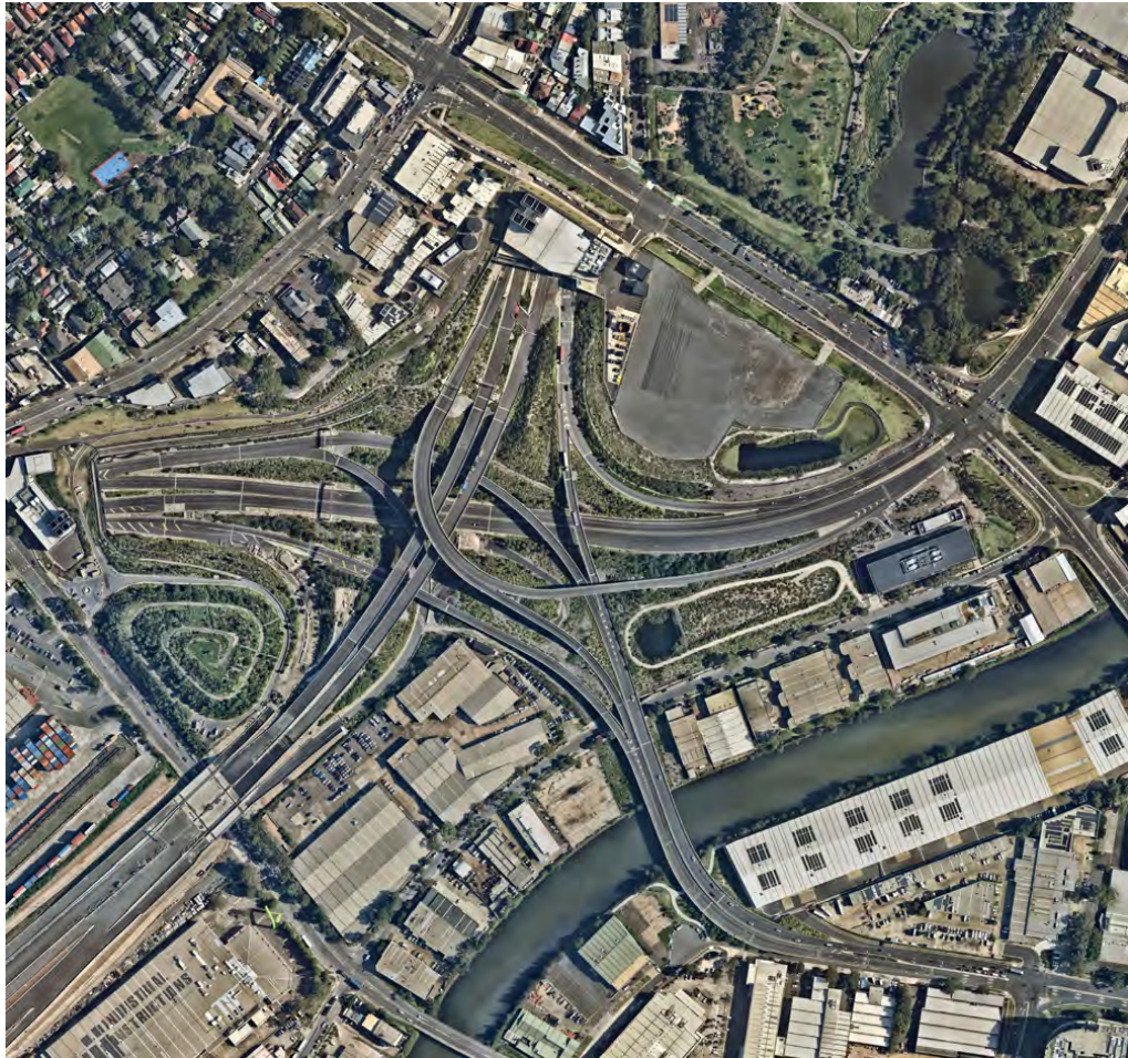
Figure 2-6 St Peters Interchange 2023 Aerial Imagery Showing Major Motorway Interchange Site near Completion (Source: Nearmap)
