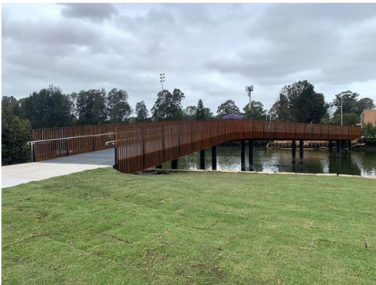
Fig 1.1 Lang Road Bridge-Cooks River Cycleway
