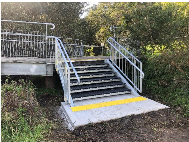
Fig 1.3 July 2024-Beaman Bridge Improvements 1 st Tee Area Marrickville Parklands.
