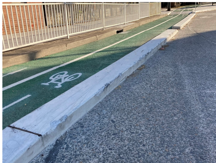
Photo 12 (Audit Finding 7) Damage to the median separating traffic from cycle lanes in Douglas St west of Percival Rd. The damage indicates numerous impacts and as well as improving delineation by use of RRPMS, a review of the turning guidelines for larger right turning vehicles (e.g. buses) from Percival Rd is suggested.
