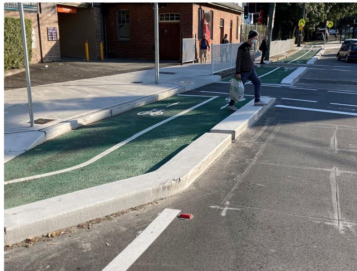
Photo 11 (Audit Finding 7) Damage to the median separating traffic from cycle lanes in Douglas St approaching Percival Rd.
