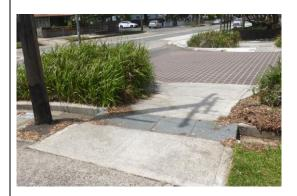
This appears to occur at pedestrian grates already in place prior to the cycleway works and these can be retrofitted with new pedestrian grates to alleviate the issue.
