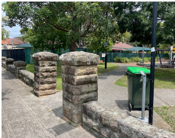
Stone wall at entrance from Malakoff Street in good condition. Preschool behind. Source Taylor Brammer Landscape Architects
