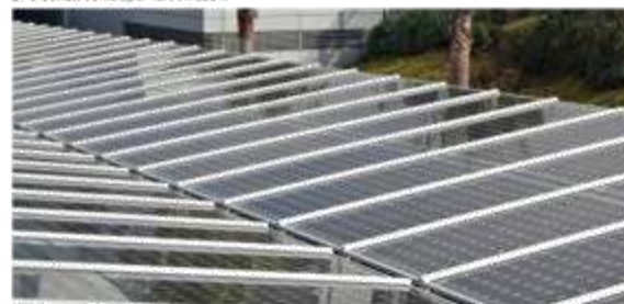
Photovoltaic solar shading structure to car park. 5
