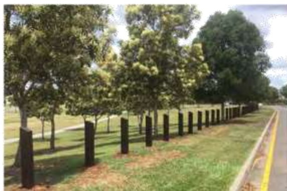
Timber bollard boundary fence type
