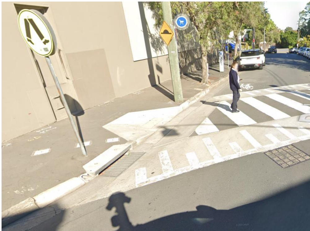
Figure 2 – raised pedestrian crossing without gutter crossing to allow for heavy vehicle swept path
